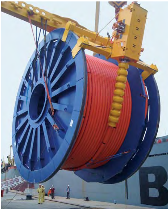
An umbilical cable on a drum ready to be placed on a ship for laying.
